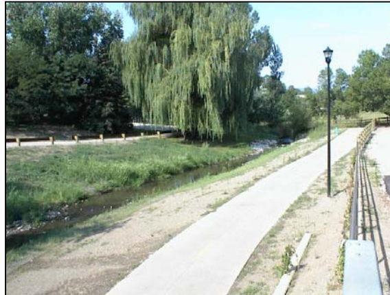
Spring Creek Channel restoration near Lemay Avenue, Fort Collins, Colorado
