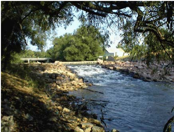
Poudre River Boat Chute/Drop Structure, Fort Collins, Colorado
