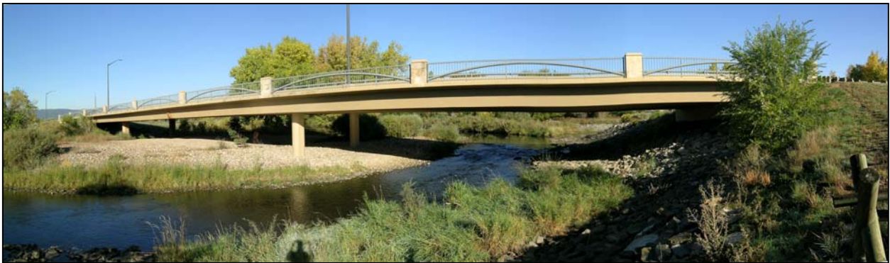
Timberline Road/Cache La Poudre River Bridge, Fort Collins, CO
