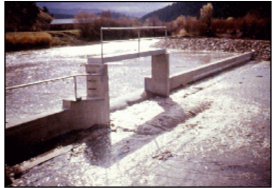
Etna Diversion Structure Salt River, Wyoming
