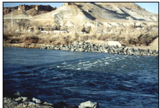
Green River Municipal Intake Structure, Green River, Wyoming
