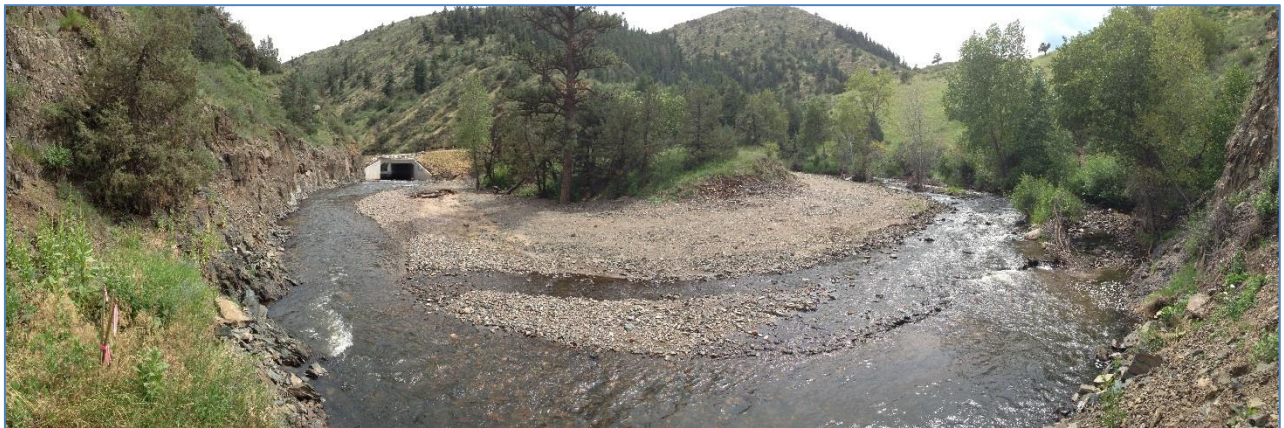
The Narrows of Larimer County Road 27 and Buckhorn Creek – Post-construction (July 2015)
