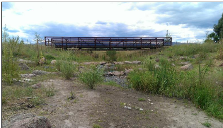
Poudre River Trail Relocation and Pedestrian Bridge Over the Outfall Channel
