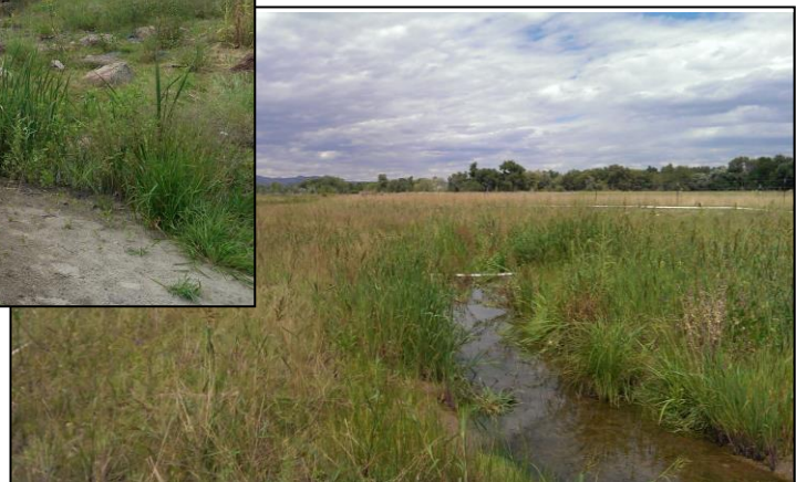
Completed Outfall Channel with Low Flow/Wetland
