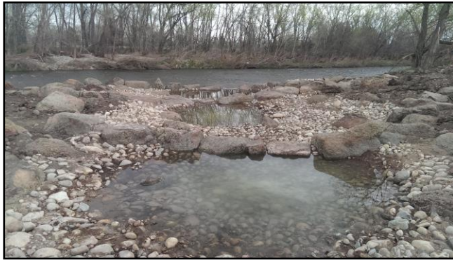
Outfall Structure at Confluence with Cache la Poudre River (Post Construction)
