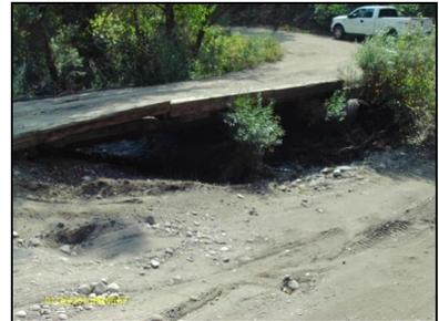
For Rist Canyon in Larimer County, eight crossings of Larimer County Road 52E (LCR 52E) were determined to be insufficient for conveying anticipated post-fire flow events. ACE **analyzed the hydraulics** associated with a 25-year flow event to **design upgrades to the existing culvert infrastructure** and to **design erosion countermeasures** for the new culvert crossings.
