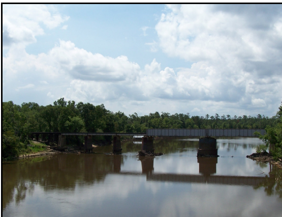
CN Railroad Crossing - Main Channel of Pascagoula River
