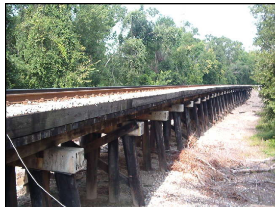
Standard Timber Ballast Deck Trestle Bridge on the CN Railroad
