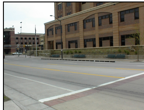
Howes Street Outfall Inlets along Laporte Avenue
