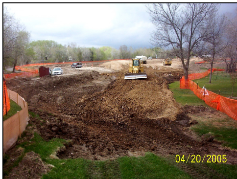
Levee During Construction
