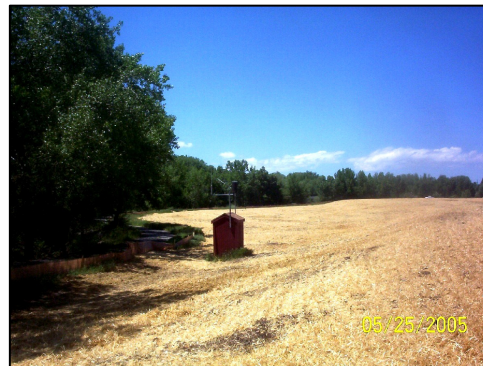
Completed Levee after Construction
