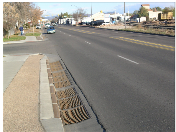
New Combination Inlets at Riverside Avenue and Whedbee Street
