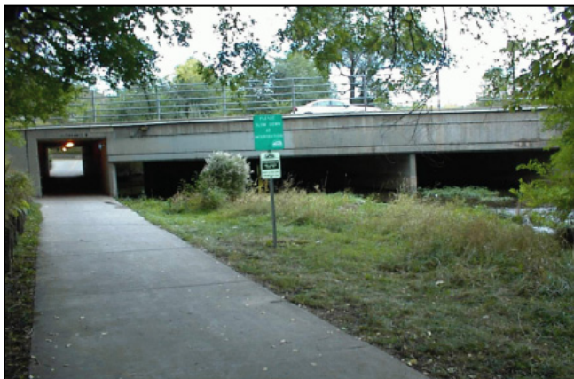
Downstream Face of Shields Street Bridge
