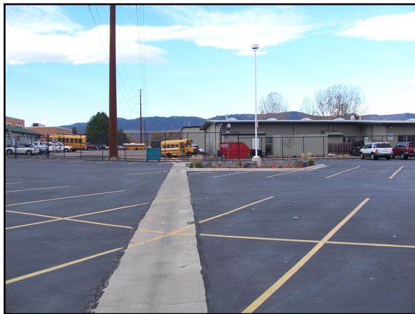
Admin Building Parking Lot Drainage Improvements
