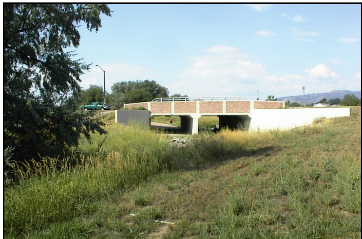
Centre Avenue Bridge at Spring Creek, Fort Collins, Colorado
