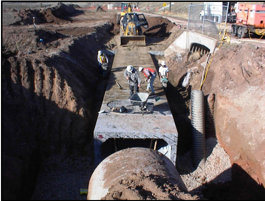
Storm Sewer Construction
