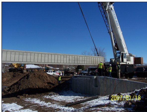
Installation of the 60 foot long flood control girder at pond outlet.
