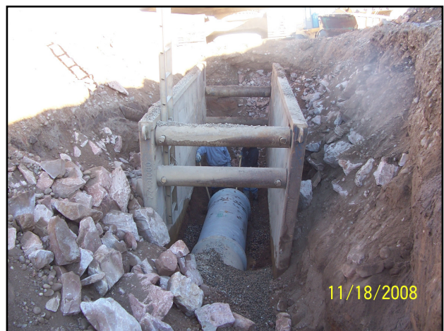
Installation of 24-inch RCP
