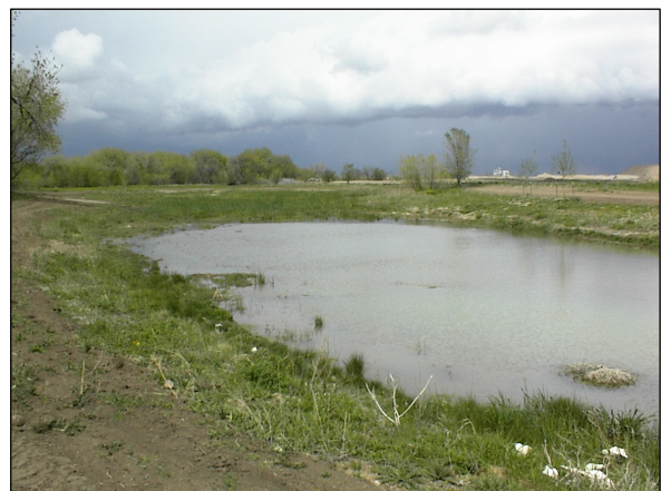
West Side Storm Sewer Wetlands Post Construction
