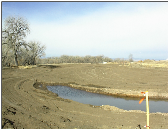
West Side Storm Sewer Wetlands During Construction
