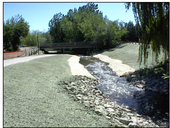
Looking Downstream from Left Bank.
