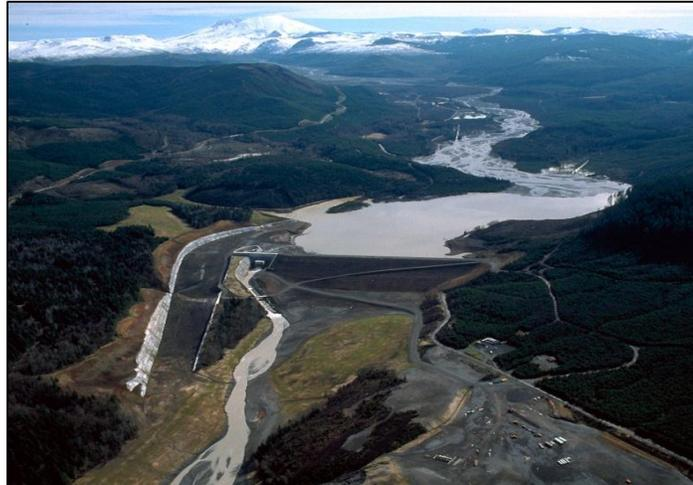
**Sediment Retention Structure (SRS)
