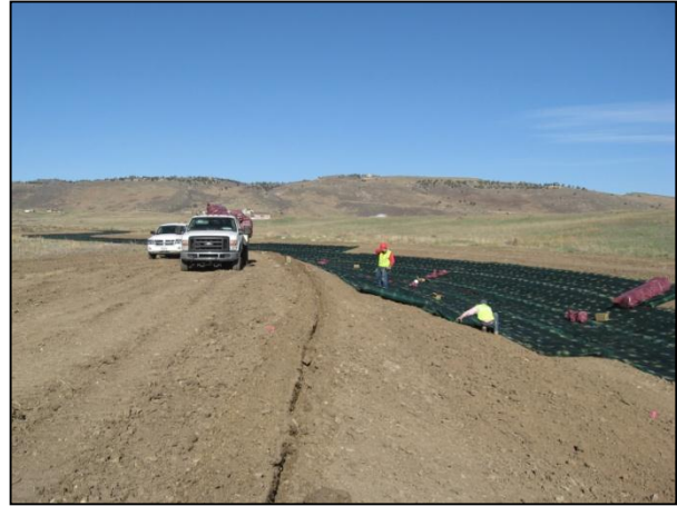
Turf Reinforcement Mat Installation
