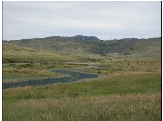
Completed Channel Realignment
